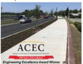
Redevelopment project which took place along US 21 Beaufort County, South Carolina. It also consisted of improvements such as the addition of a raised median, construction of a multi-use path, landscaping, lighting, signal work, and undergrounding of existing overhead utilities.
